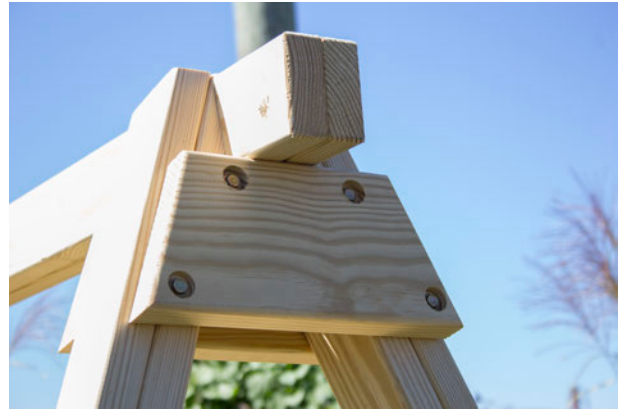
Top Brace connection shown
