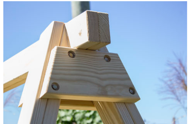
Top Brace connection shown
